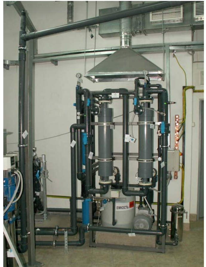
Liqui-Cel® Water Degassing System used at the Ice Palace to produce Crystal clear ice at the arena
